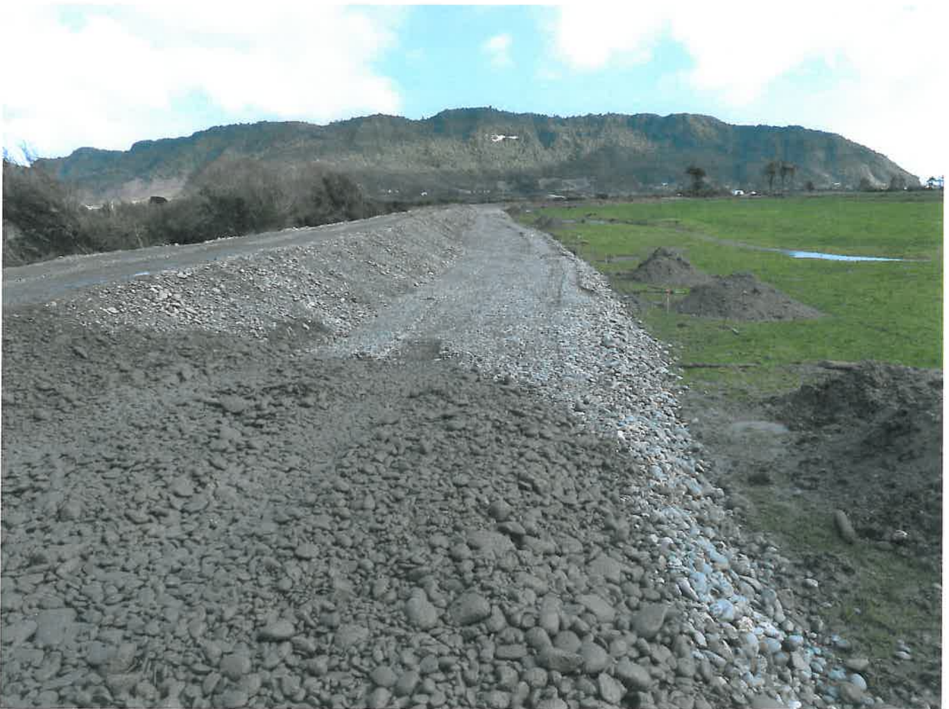
Coal Creek stopbank upgrade in progress
